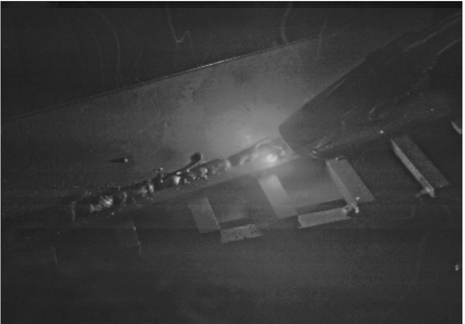
Figure 2: Welding scene view using TEREBES welding helmet. Courtesy: Hillers, Aiteanu [6].
