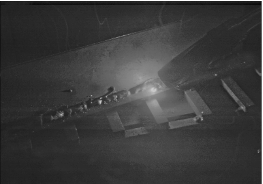
Figure 2: Welding scene view using TEREDES welding helmet. Courtesy: Hillers, Aiteanu [6].
